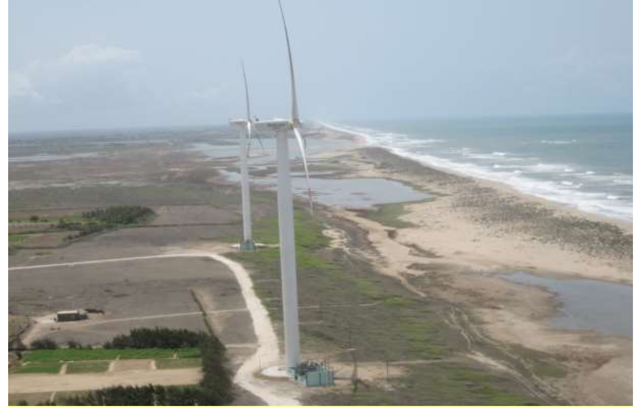
Wind Power Plant
