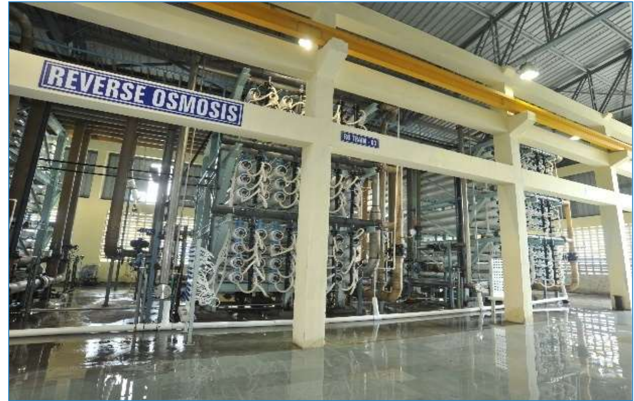
Tertiary Treatment Plant
