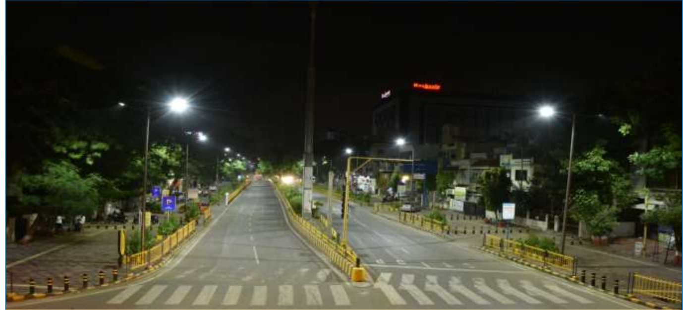
LED Street Lights
