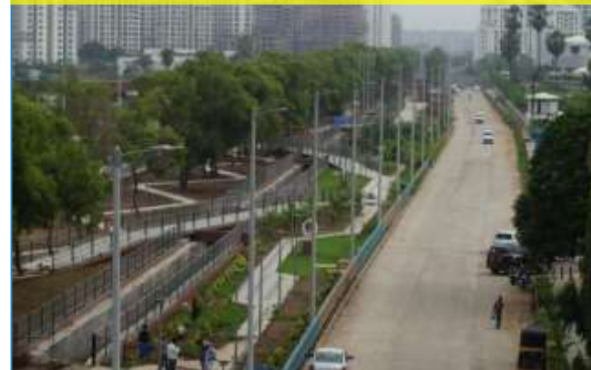
Canal Road Re-Development
