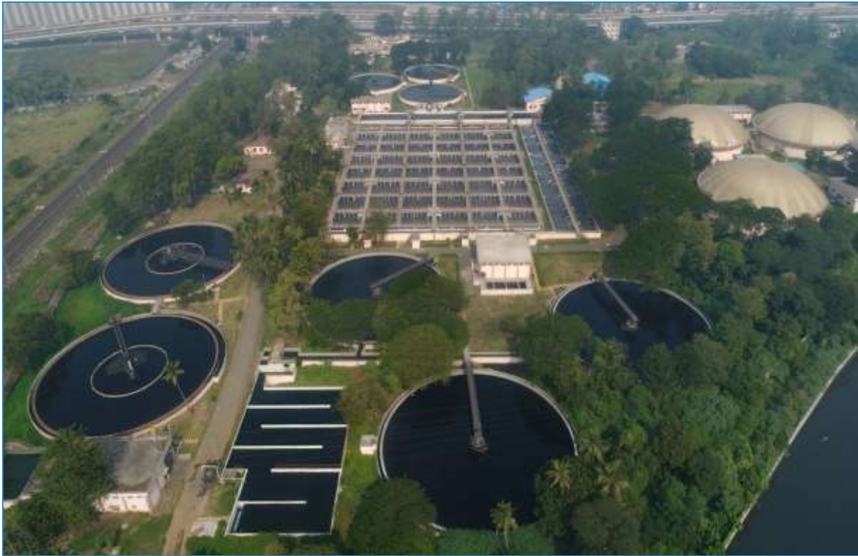
Sewage Treatment Plant with SCADA & Energy Generation
